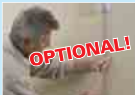
7.) Fix cable with the transparent cable duct.
