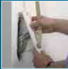
2: Disassemble old belt winder.
