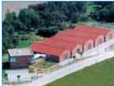
Premises in Dresden
